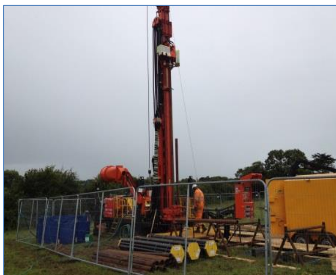
Figure 1 Priority Drilling Operating the Hanjin D&B35 Rig
